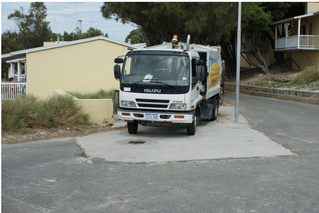
Figure C6 Road drain at Longreach Bay, photograph by C. Loos
