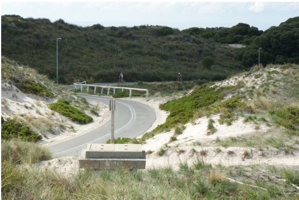
Figure C12 Vents for sewer pump stations and sealed roads in Longreach Bay saltwater bore field, photograph by C. Loos
