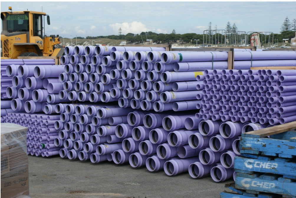
Figure C10 Pipes for treated wastewater for proposed use at the island's golf course, photograph by C. Loos
