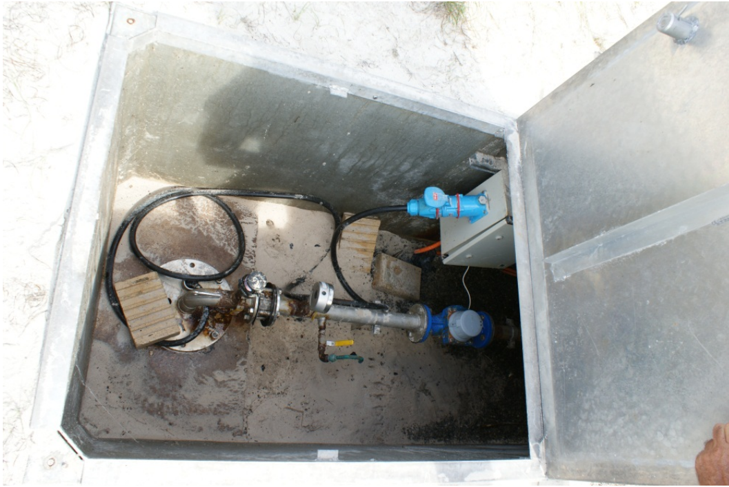
Figure C3 Bore compound for saltwater bore at Longreach Bay, photograph by C. Loos
