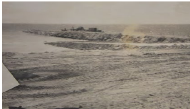
Plate 6: Reconstruction works, rockfill and barge hardstand (NAA)
