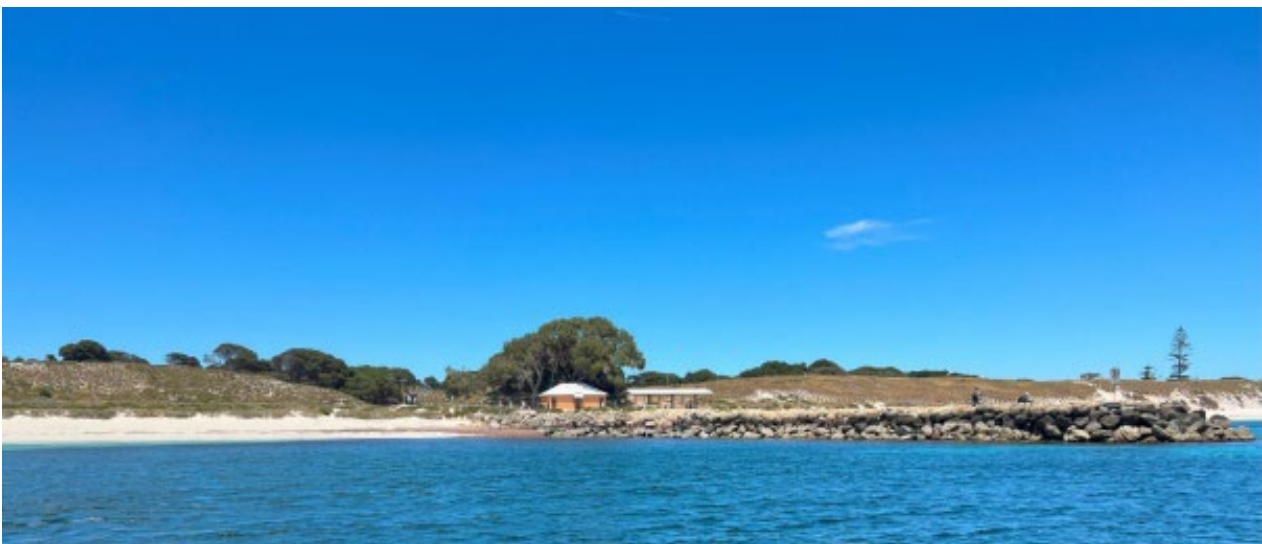
Plate 10: Army Groyne structure with a view of Thomson Bay to the west and view of the groyne from the eastern seaward side
