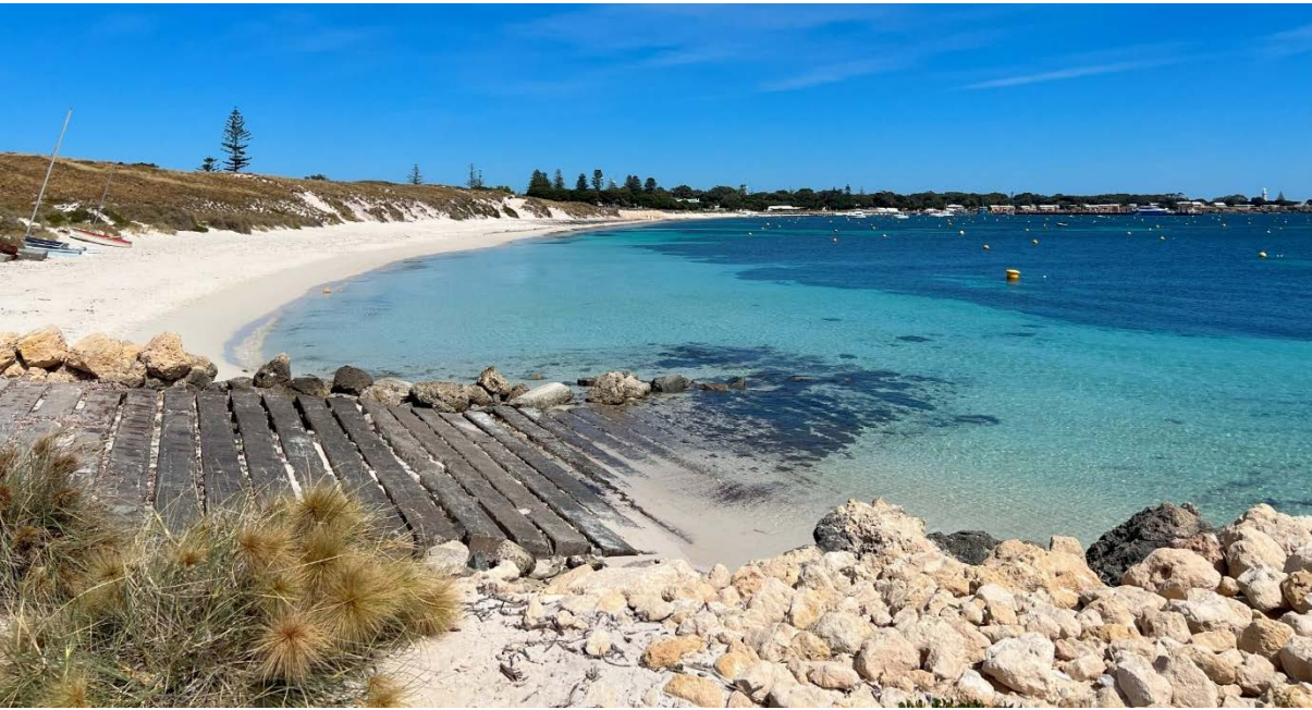
Figure 1.4: View of Thomson Bay to the west of the Army Groyne structure
