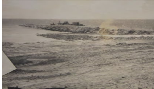
Plate 6 Reconstruction works, rockfill and barge hardstand (NAA)
