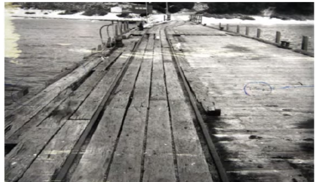
Plate 4 Original timber jetty facing west to shore (National Archives Australia (NAA))
