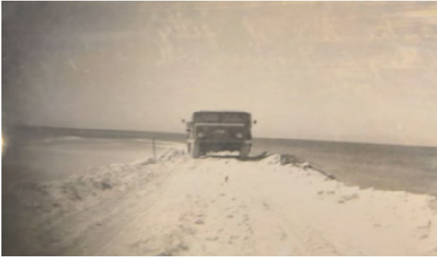
Plate 5 Reconstruction works, 1971 (NAA)
