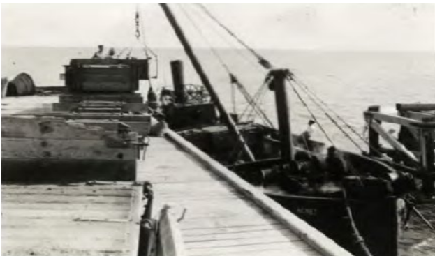
Plate 3 Original timber jetty with gantry on the right, facing west (RIA 2012.265)
