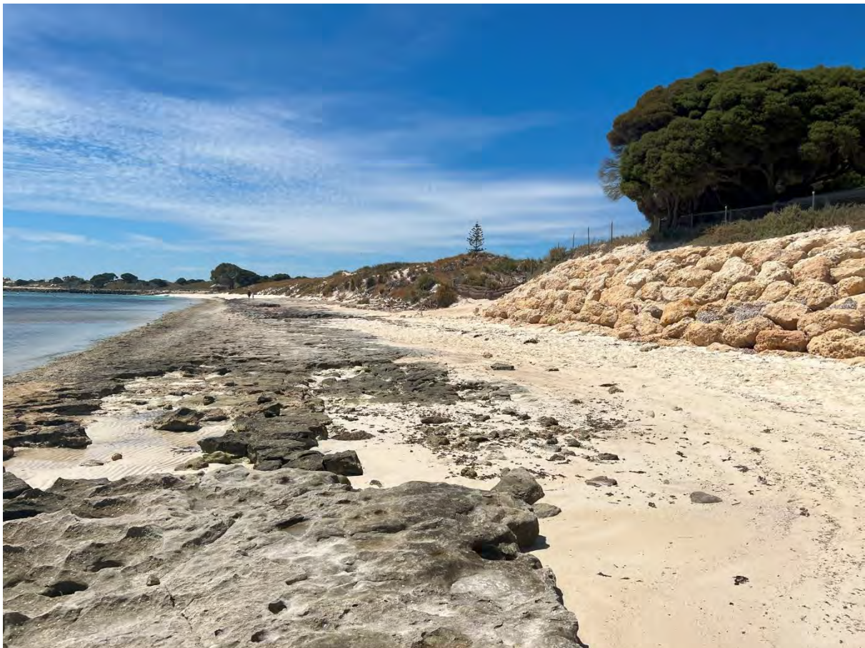
Figure 2.15: Rock pavement/platform supporting the perched beaches of Thomson Bay, as seen in front of the South Thomson Bay seawall.
