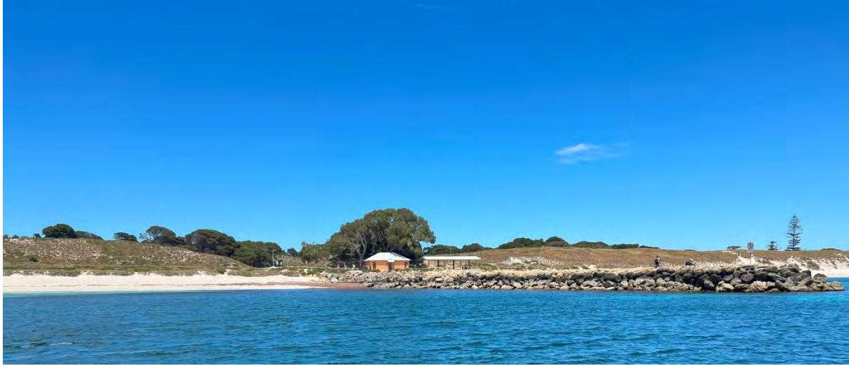
Figure 2.14: View towards the Army Groyne structure, showing dune height east and west of the structure
